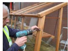
The roof panel should be installed on every timber support. You should fix these two components using stainless steel screws.
